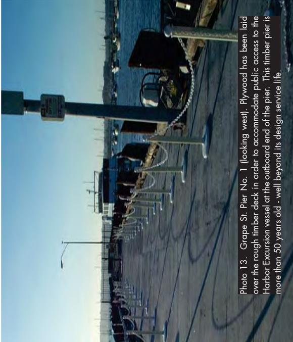
Photo 13. Grape St. Pier No. 1 (looking west). Plywood has been laid over the rough timber deck in order to accommodate public access to the Harbor Excursion vessel at the outboard end of the pier. This timber pier is more than 50 years old - well beyond its design service life.
