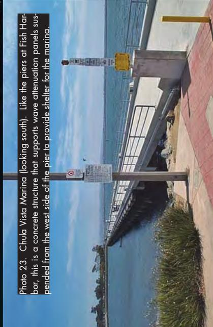
Photo 23. Chula Vista Marina (looking south). Like the piers at Fish Harbor, this is a concrete structure that supports wave attenuation panels suspended from the west side of the pier to provide shelter for the marina.
