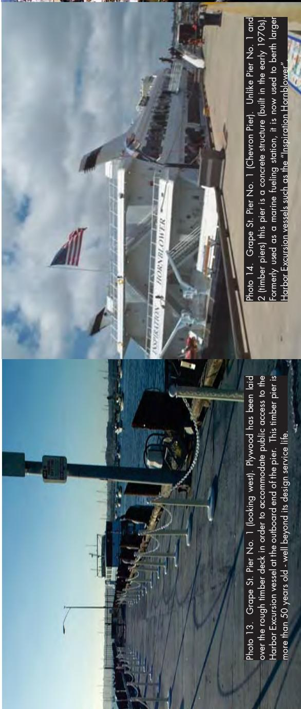
Photo 13. Grape St. Pier No. 1 (looking west). Plywood has been laid over the rough timber deck in order to accommodate public access to the Harbor Excursion vessel at the outboard end of the pier. This timber pier is more than 50 years old - well beyond its design service life.
