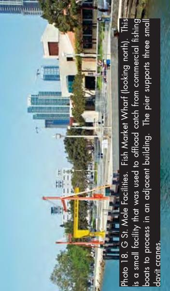
Photo 18. G St. Mole Facilities. Fish Market Wharf (looking north). This is a small facility that was used to offload catch from commercial fishing boats to process in an adjacent building. The pier supports three small davit cranes.
