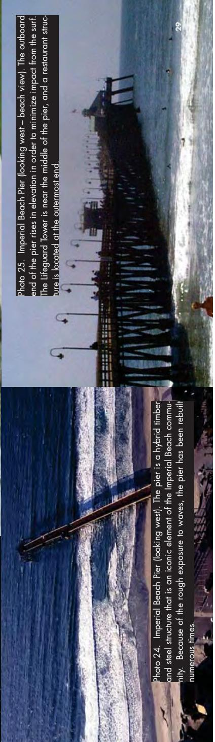
Photo 24. Imperial Beach Pier (looking west). The pier is a hybrid timber and steel structure that is an iconic element of the Imperial Beach community. Because of the rough exposure to waves, the pier has been rebuilt numerous times.
