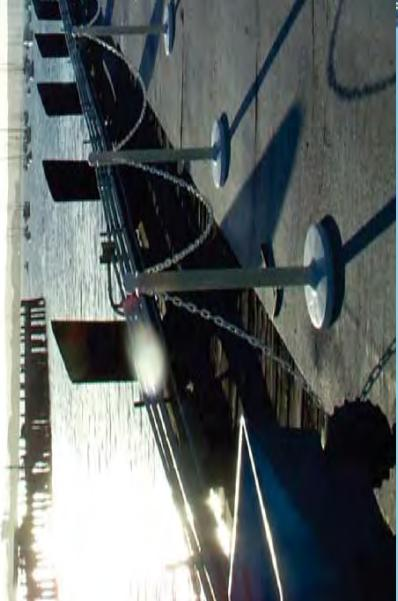
Photo 12. Grape St. Piers (looking east). Pier Nos. 1 and 2 are timber structures in poor condition - formerly used to support the San Diego tuna fleet. Pier No. 3 on the right will was formerly known as "Chevron Pier".
