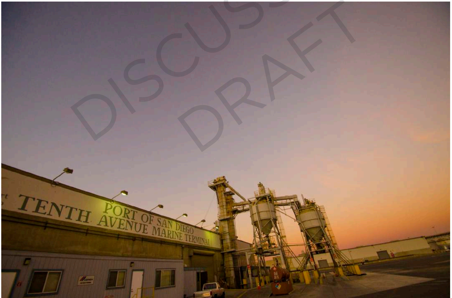
Tenth Avenue Marine Terminal
