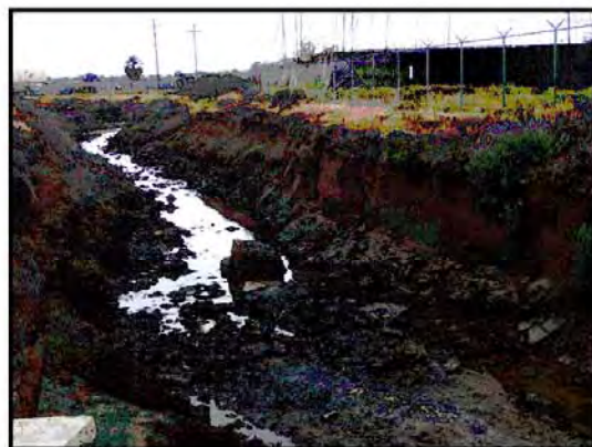
Looking east at the steeply sloped entrance channel. Concrete rubble is visible and the channel is eroding as it widens over time.
