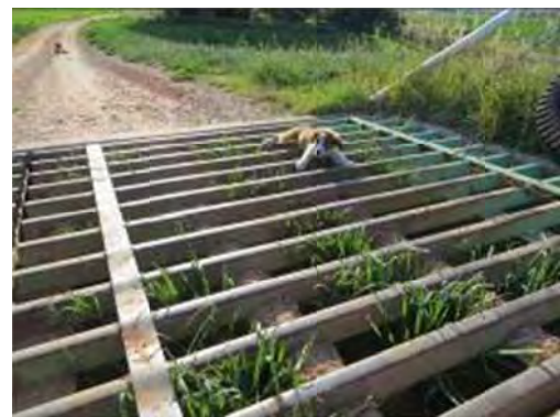
Example of a bridge crossing (top) and box culvert with cattle guard (bottom) that could be used to control predators and provide a marsh connection along the CVWR access road.
