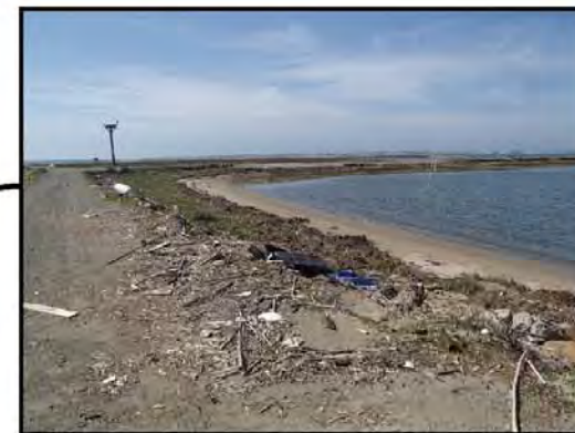
Looking west along the same portion of roadway. Presence of marine wrack is indicative of overtopping of the dike/roadway during king tides.
