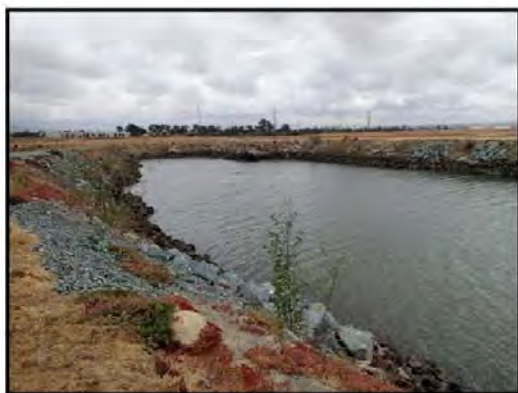
Looking east at the terminus of discharge channel basin. A storm drain enters the south side of the basin at the toe of the rip rap.
