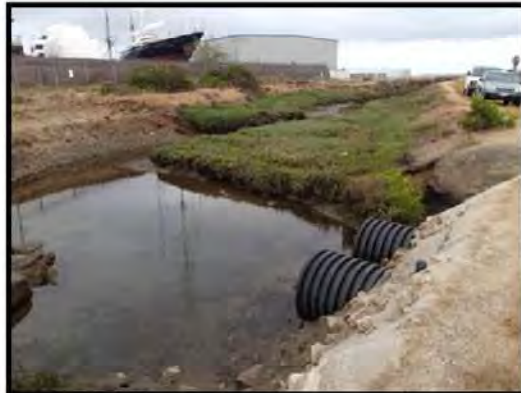
Twin 24-inch corrugated drains bring tidal waters to the F&G Street Marsh via a narrow entrance channel
