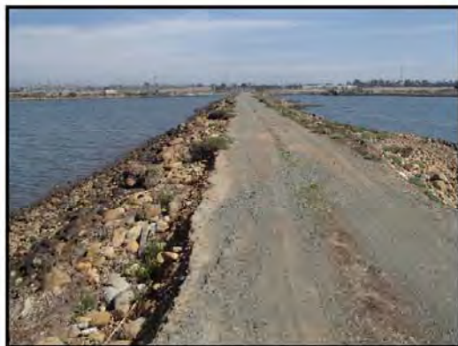
Looking east toward the decommissioned SBPP along the constructed dike that serves at the roadway access to CVWR. The roadbed is not uniformly armored and is eroding.
