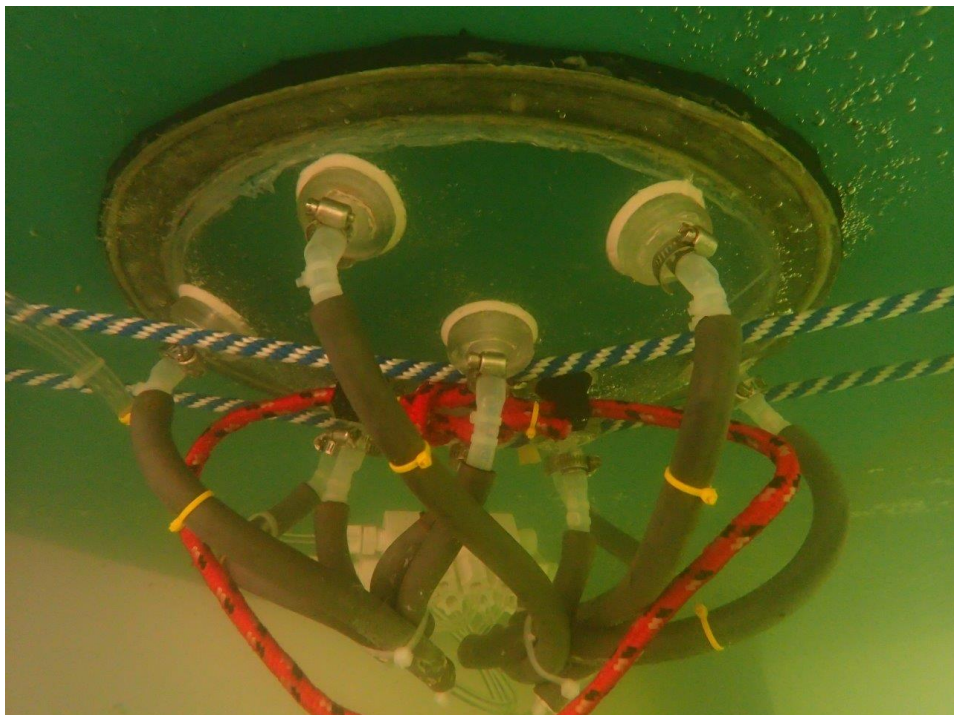
Figure 2-6. Fully installed dome during sampling operations.
