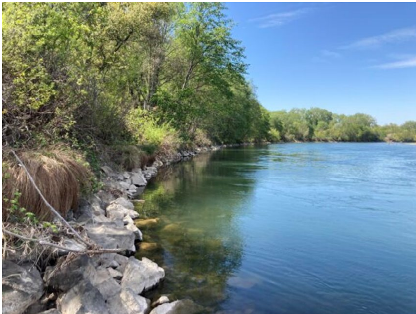
Kopta Slough: Kopta Slough Multi-Benefit Project. Photo source: California Department of Water Resources / acceleratingrestoration.org
