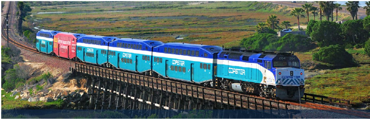
LOSSAN Corridor, San Elijo Lagoon: Photo of the LOSSAN rail corridor running alongside San Elijo Lagoon, with an Amtrak Coaster train on the tracks.
