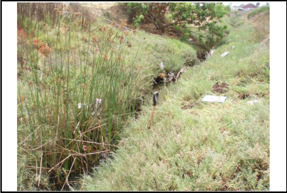
Photo Point 71. Data point 71 is located along the inside edge of the bottom of the channel that defines the eastern limits of the study area, immediately east of DP 70. Photo is directed south and was taken July 7, 2008.
