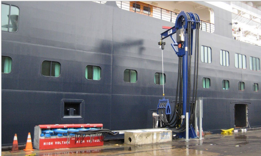
Figure IV.6-1 Street Cruise Ship Terminal Shore Power System 9
