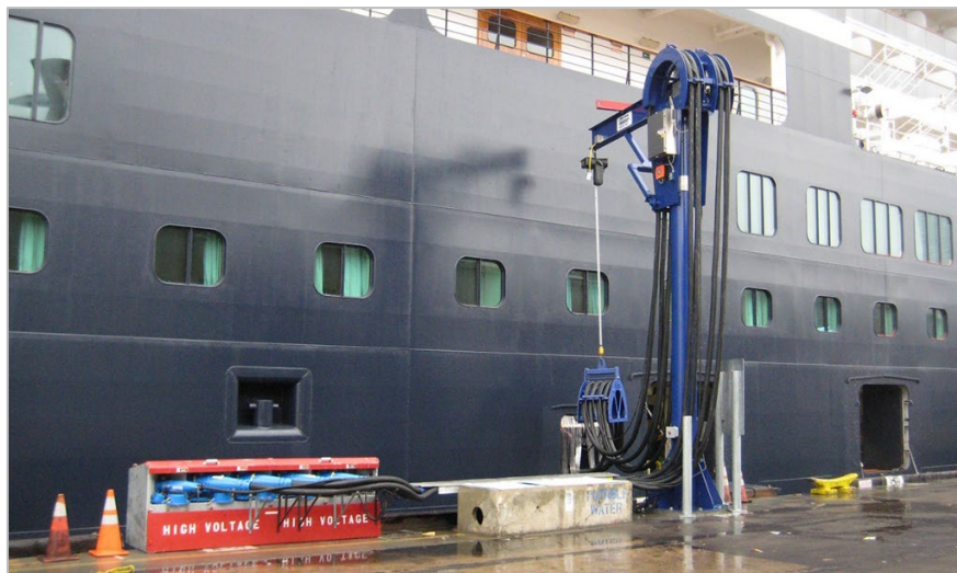
Figure IV.6-1 Street Cruise Ship Terminal Shore Power System 9
