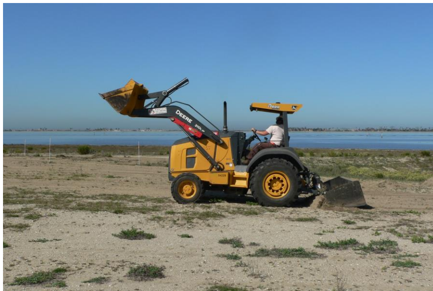
Mechanical scraping to reduce vegetation and prepare the site for least tern nesting.
