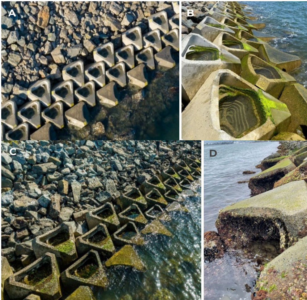
Figure 7- The biological growth covering the CL over time. (A) The CL on the day of deployment, (B) three MPD, (C) 14 MPD, and (D) 26 MPD.
