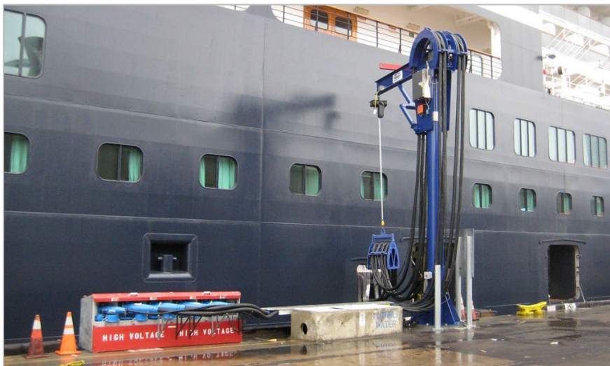
Figure IV.6-1 Street Cruise Ship Terminal Shore Power System 9
