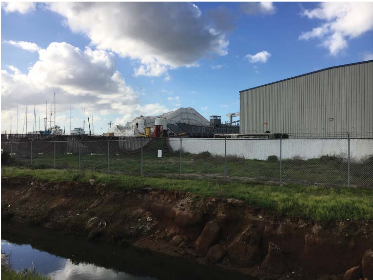
Figure 1-3: Photos of Existing Channel
