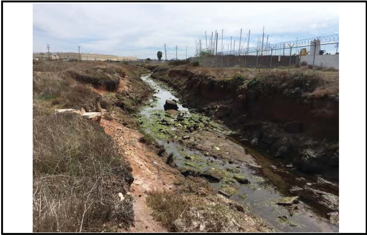
Photo 1. Overview photo; taken from the western portion of the BSA and directed southeast. Photo taken on 3/9/2018.
