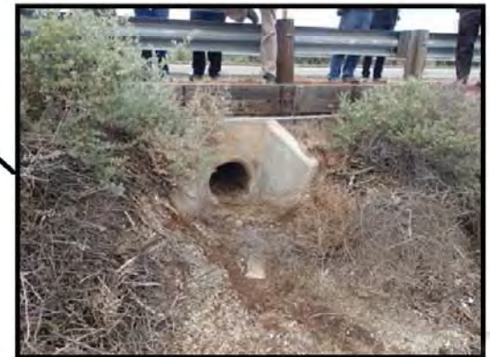
An 18-inch concrete culvert connects F&G Street Marsh to the Seasonal Wetlands beneath Lagoon Drive
