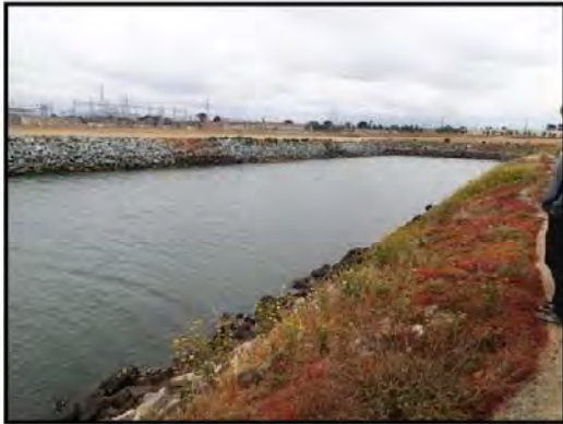
Looking east at the terminus of the intake channel basin. A storm drain enters the north side of the basin midway down the rip rap.
