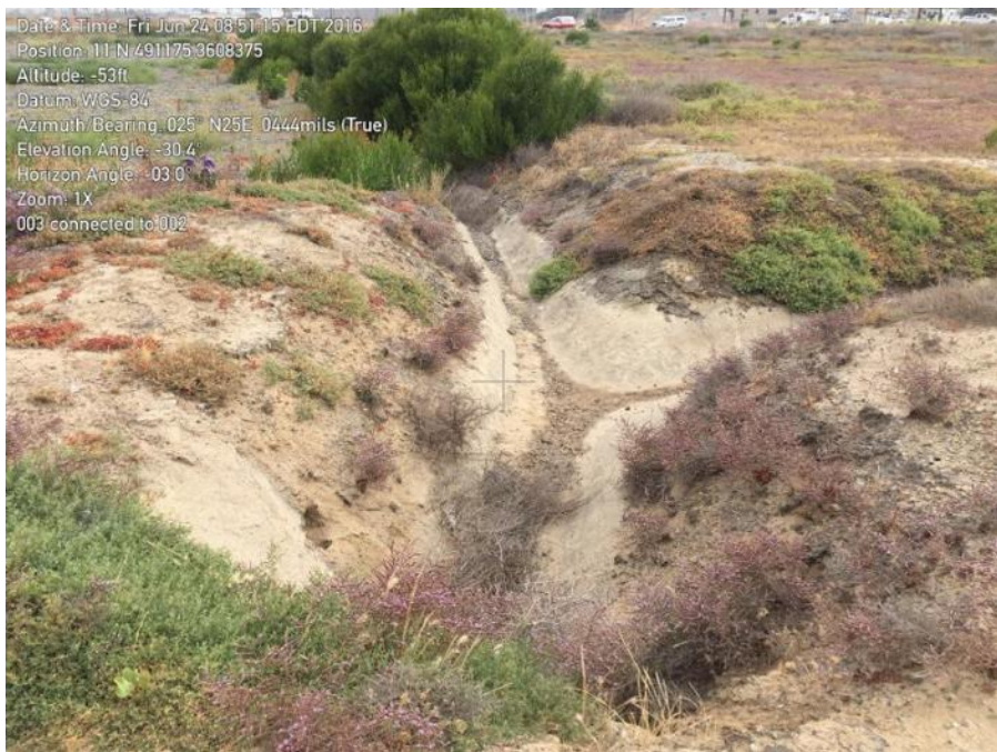
Photo Point 16: Drainage ditch
