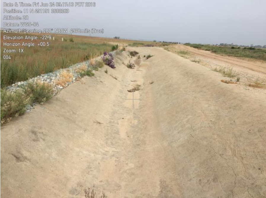
Photo Point 19: Drainage ditch
