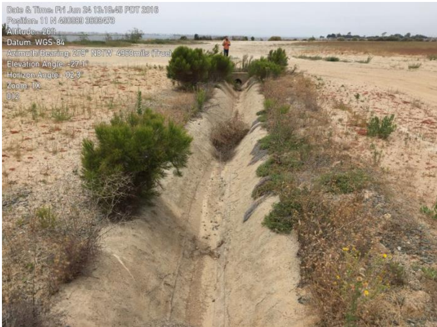
Photo Point 12: Drainage ditch
