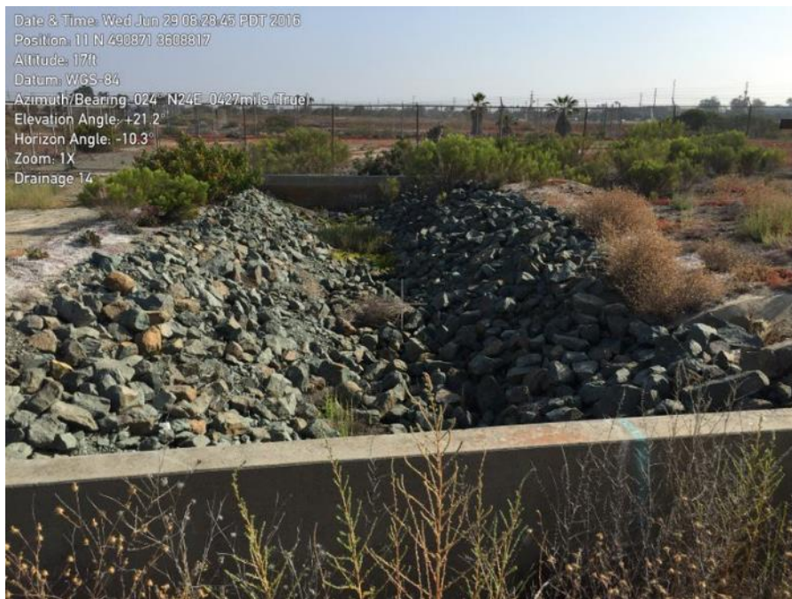
Photo Point 6: Drainage ditch
