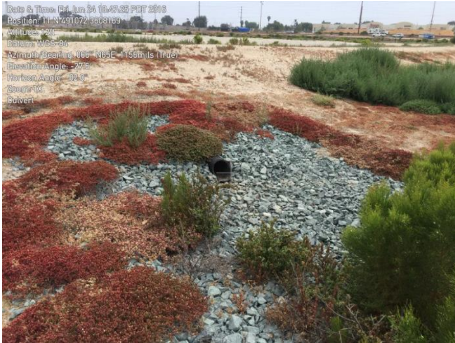
Photo Point 30: Culvert to drainage ditch
