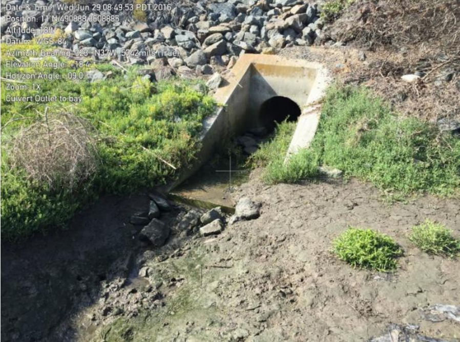
Photo Point 3: Culvert out to San Diego Bay
