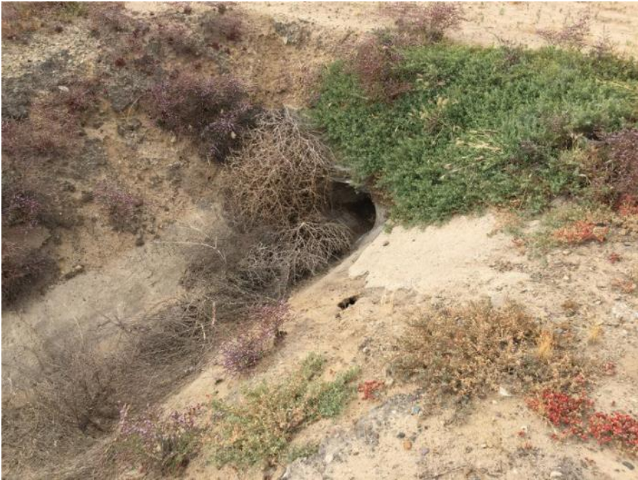
Photo Point 18: Culvert to drainage ditch
