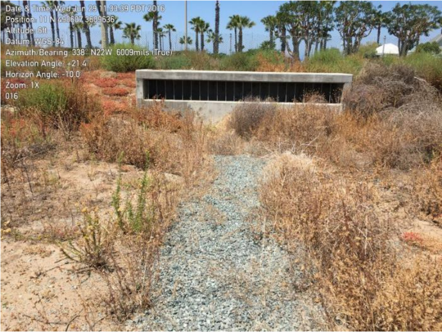
Photo Point 1: Drainage ditch leading to box culvert
