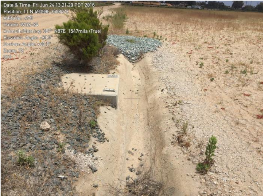
Photo Point 11: Drainage ditch
