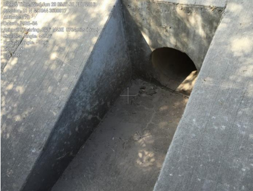
Photo Point 5: Culvert to drainage ditch with freshwater marsh vegetation
