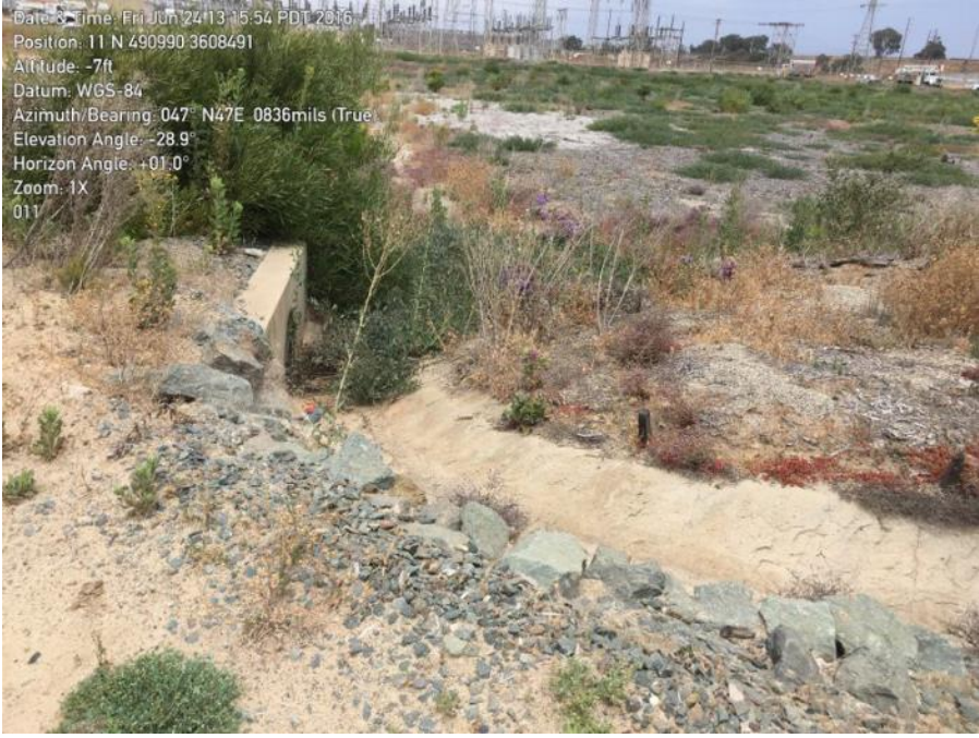
Photo Point 10: Drainage ditch
