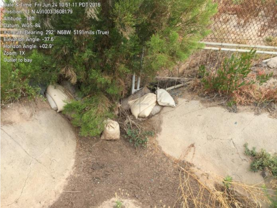
Photo Point 29: Drainage ditch outlet to San Diego Bay
