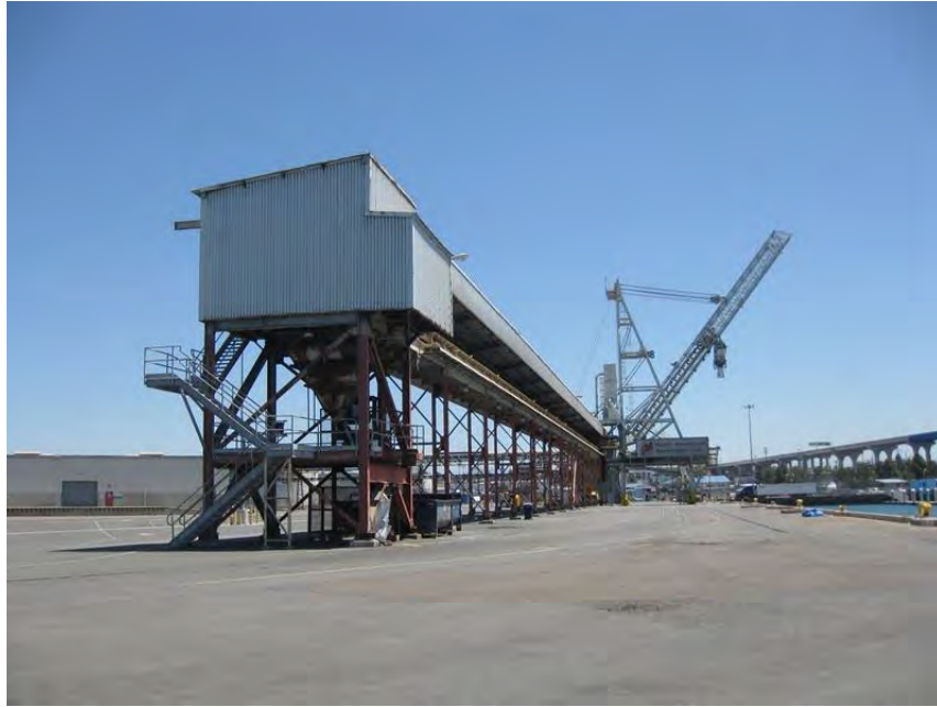
Photograph 8: Southern end of bulk loader system, including elevated conveyor, corrugated metal conveyor shelter, and traveling loader with telescoping chute (center-right background), looking east-southeast
