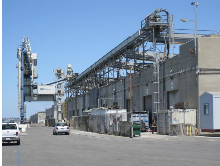
Figure 18. Non original cement unloading and conveyance facilities at south end of southeast elevation, looking north-northwest
