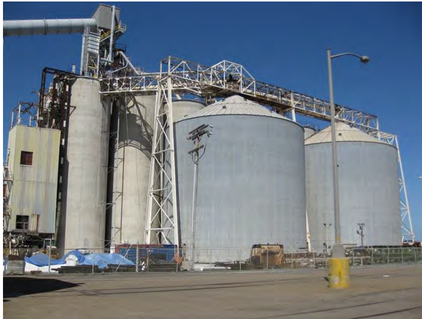
Photograph 2: Northeast side of silo cluster, note two larger silos constructed since the 1970s, and multistory corrugated-metal structure (far left) that appears to have been built with the larger silos. Also note elevated conduit and square element constructed within the past decade (upper left). Looking west-southwest
