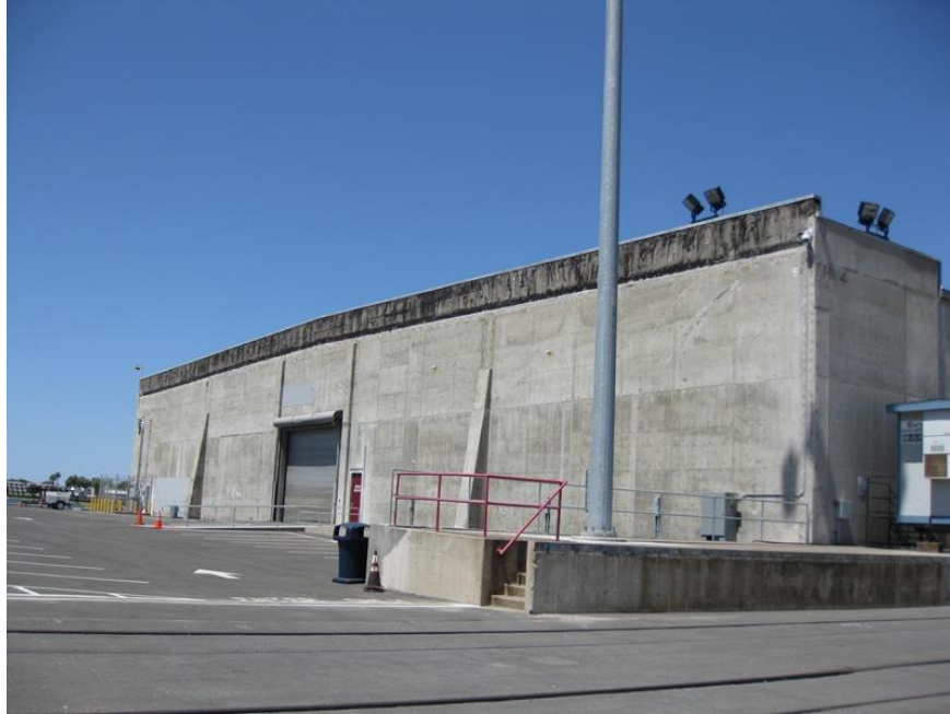
Figure 14. Former interior concrete wall that now forms the southwest elevation of Transit Shed #1, which faces Transit Shed #2's surviving headhouse; note partially remaining "Berth 4" signage (upper right) indicating extent of demolition at southern end of building, looking west
