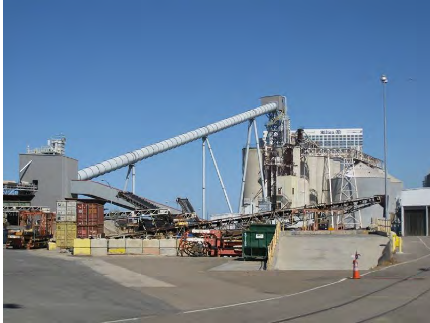
Photograph 6: View highlighting elements of bulk loader system added within the past decade, including recent junction structure and conduit four-sided conduit connecting to original junction house (dark gray, left), and elevated cylindrical conduit extending from the top of the silo complex to the recently constructed junction structure. The steel conveyor apparatuses between the aforementioned features and the concrete ramp at the right are also elements of the system introduced after 1970, looking north-northwest.
