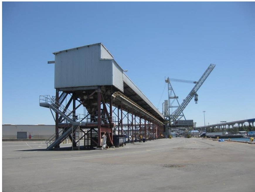
Figure 24. Southern segment of bulk loader system, including elevated conveyor, corrugated metal conveyor shelter, and traveling loader with telescoping chute (center-right background), looking east-southeast
