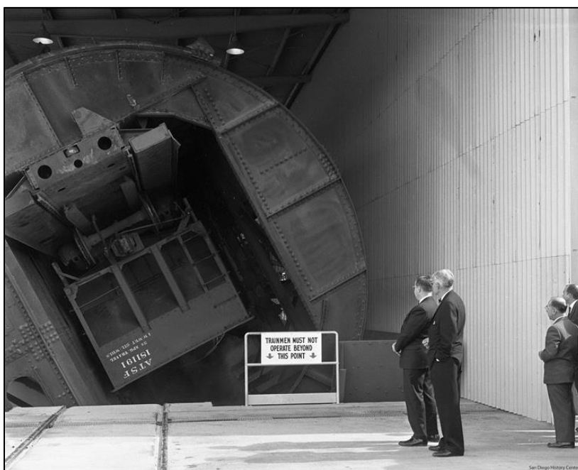
Figure 11. Demonstration of rail car unloader during 1963 dedication of the Tenth Avenue Marine Terminal's bulk loader system; Port Director John Bate at far right (from San Diego History Center Photograph Collection, UT-85.D338, No. 8)
