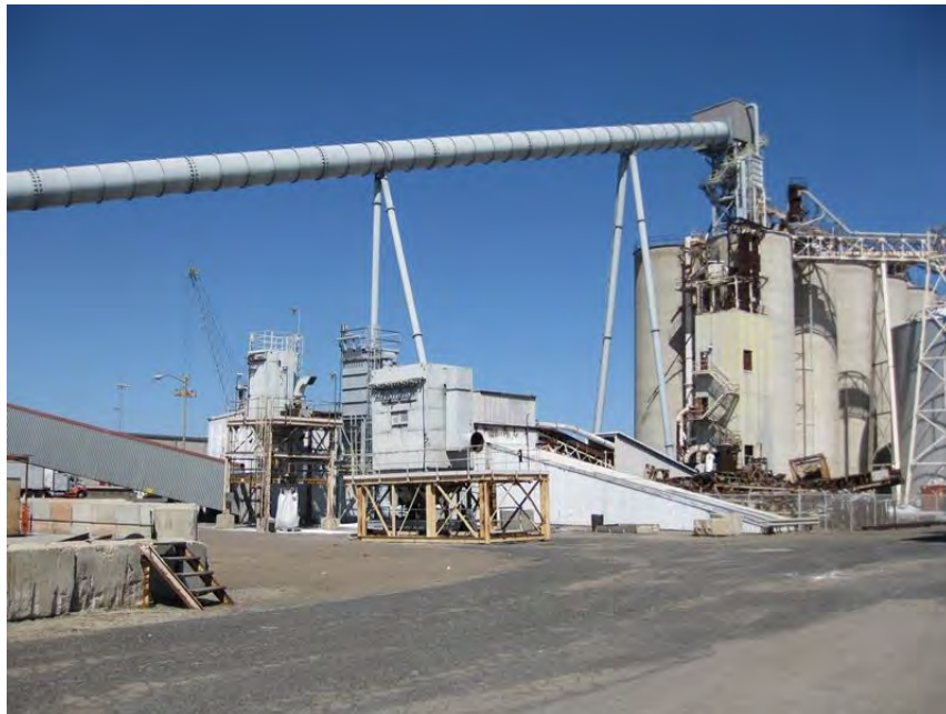
Photograph 5: Original bulk loader junction house west of rail car unloading building. Note elements constructed within the past decade, including four-sided conduit (dark gray) extending south from original junction house to recently constructed junction house, and conduit from recently constructed junction house to top of silos looking west-northwest
