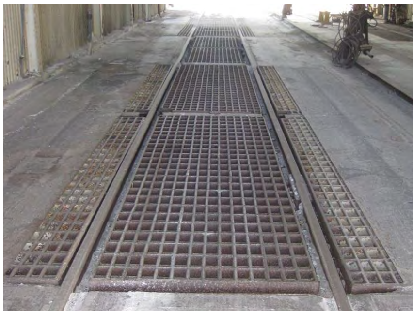
Photograph 3: Steel grills for dumping of commodities underneath rail cars within westerly enclosed portion of rail car Unloading Building, looking southeast
