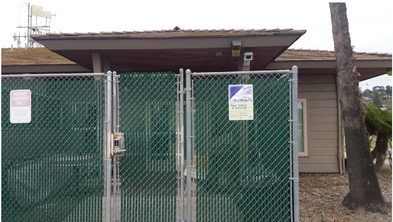
Photograph 4. LT-1: Camera facing west
