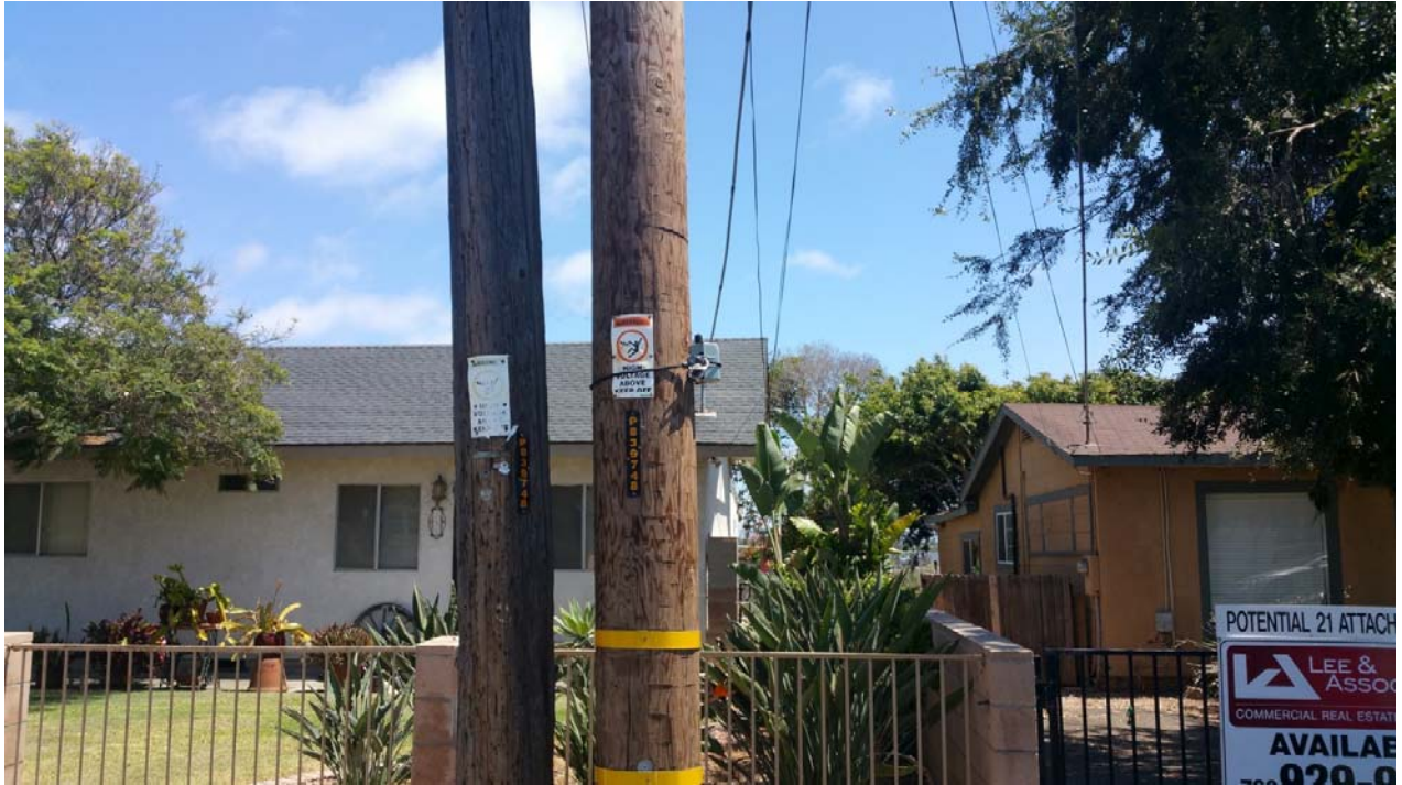
Photograph 15. LT-4: Camera facing south
