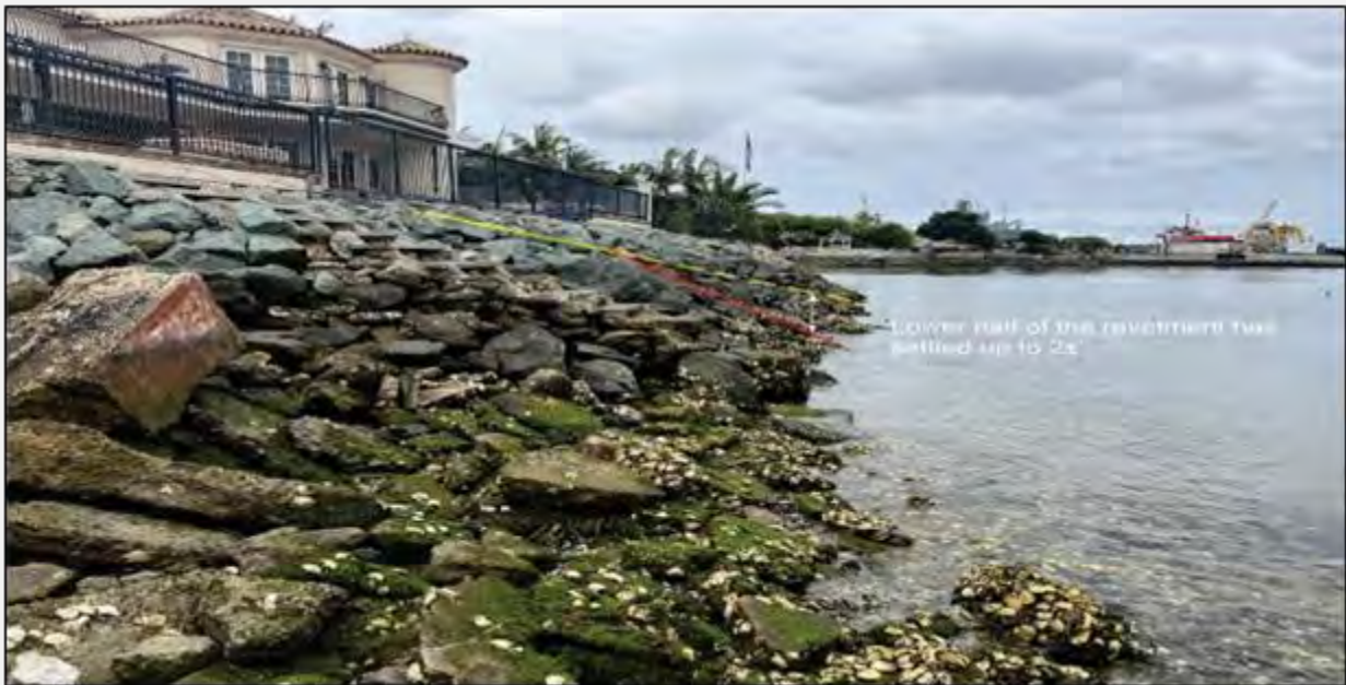
Exhibit 2-3. Existing Granitic Rock Revetment at 407 First Street
