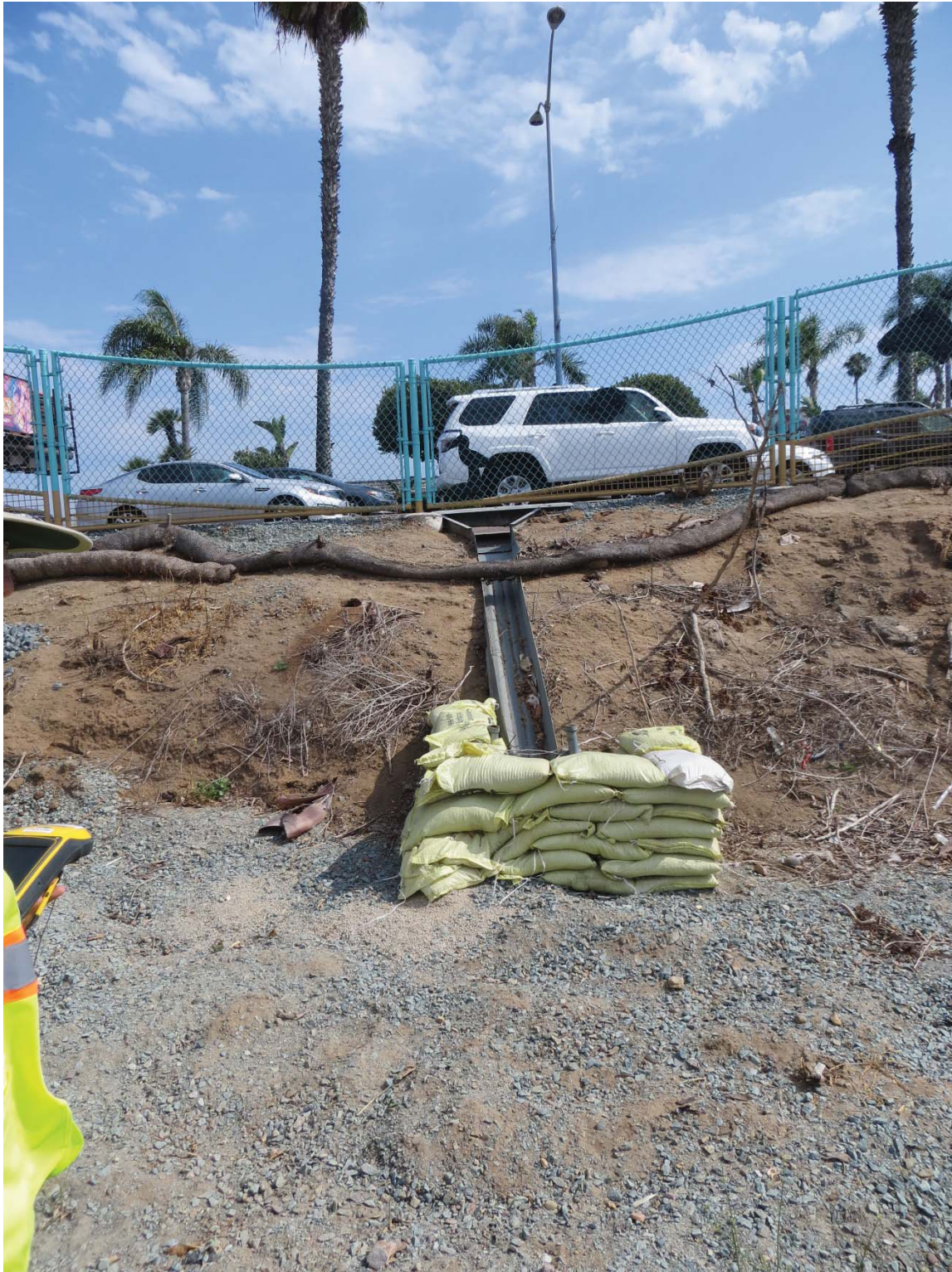
PHOTO 9: STORMWATER CONVEYANCE #1 ENTERING BERMED AREA FROM PALM AVENUE
