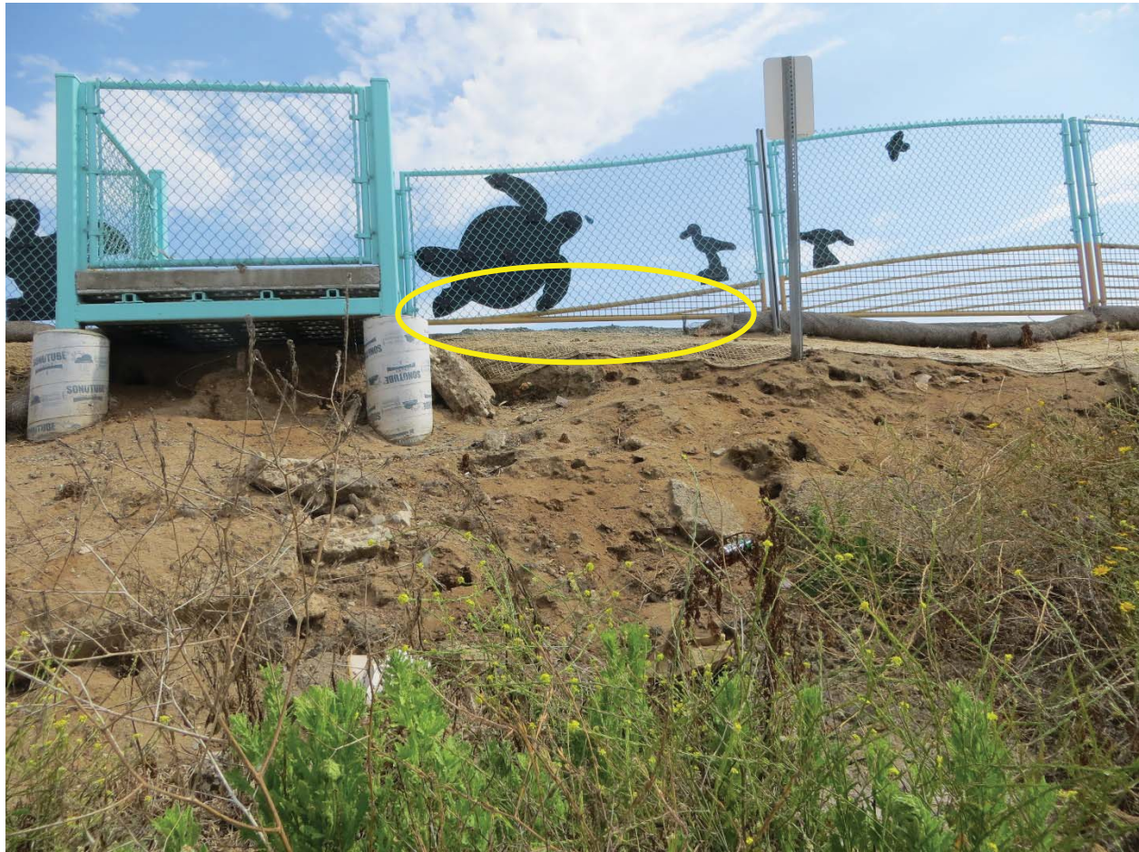
PHOTO 11: EROSIONAL GULLY CAUSED BY STORMWATER ENTERING BERMED AREA THROUGH BREAK IN WATTLES
