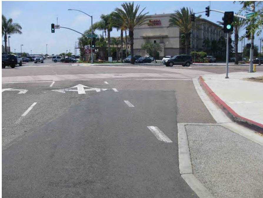
Photograph 5. Paved over section of the Coronado Belt Line approaching intersection of Cleveland Avenue and Bay Marina Drive (formerly 24th Street), where rails appear to have been removed, looking south-southwest.
