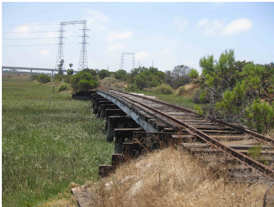
Photograph 9. Timber trestle carrying track over Paradise Creek Marsh approximately 1,600 feet north of Sweetwater River Channel, looking south-southeast.
