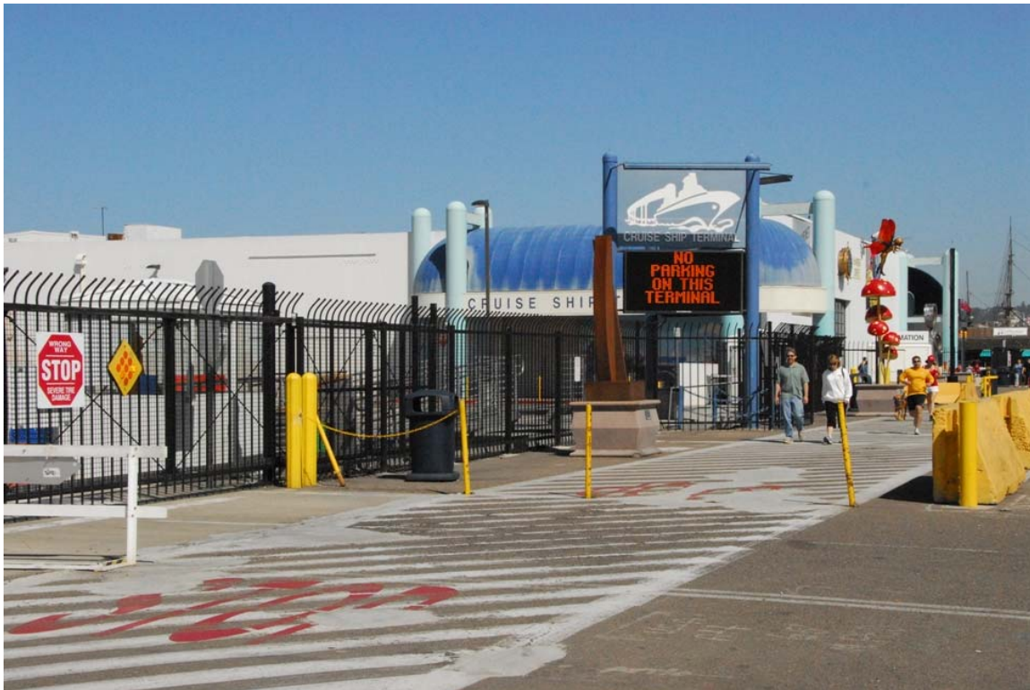
Figure 9: View of Eastern End of B Street Pier and Sign for CST (Facing Northwest)
