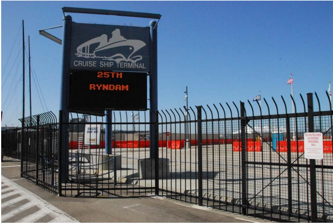
Figure 8: View of Eastern End of B Street Pier and Sign for CST (Facing Southwest)
