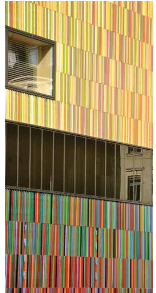
The façade of Sauerbruch Hutton's Brandhorst Museum is a brilliant example of mixing glass and non-glass materials. Photo by Tony Brady
