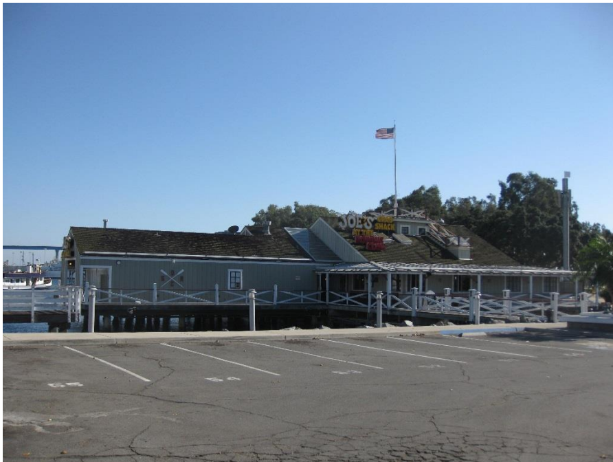
Photograph 1. View to southeast toward front of San Diego Rowing Club. October 25, 2016
