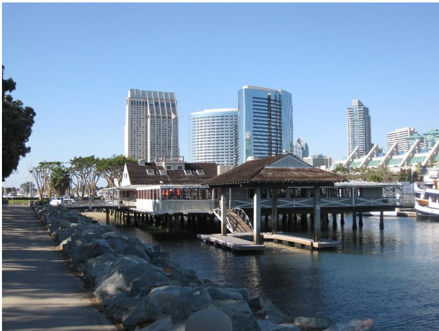
Photograph 3. View northwest toward rear of building. October 24, 2016
