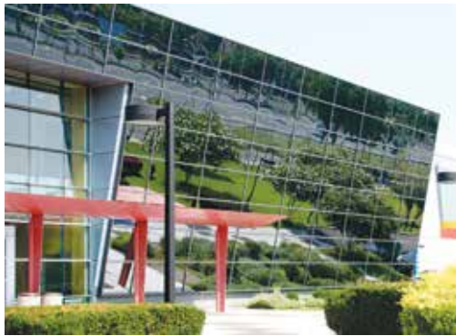
Reflections in this angled façade can be seen clearly over a long distance, and birds can approach the glass from any angle. Photo by Christine Sheppard, ABC
