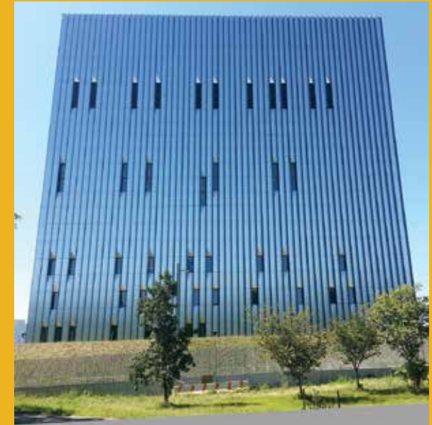
The area of glass on a façade is the strongest predictor of threat to birds. There are also other reasons to limit glass. Skidmore Owings Merrill’s Bronx, New York, Emergency Call Center is a handsome example of creative design with restricted glass, for a building intended to be both secure and blast-resistant. Photo by Chris Sheppard, ABC
