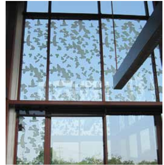
The design of the Grange Insurance Audubon Center in Columbus, Ohio, includes many panels of glass, fritted with the silhouettes of species of birds in flight. Photo by Christine Sheppard, ABC
