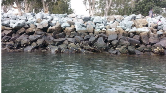
Intertidal rip-rap on the Embarcadero Marina Park South shoreline. Small white "dots" on rocks are oyster.
