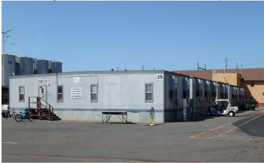
Modular offices to be removed in-way-of admin. office construction
