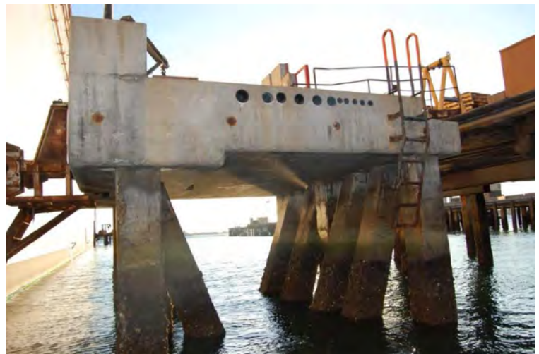
Existing Pride of San Diego dolphin to be demolished for new dolphin construction
