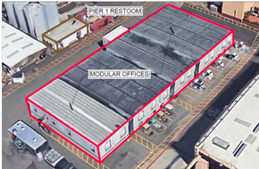
Existing modular offices footprint of new admin. office complex
