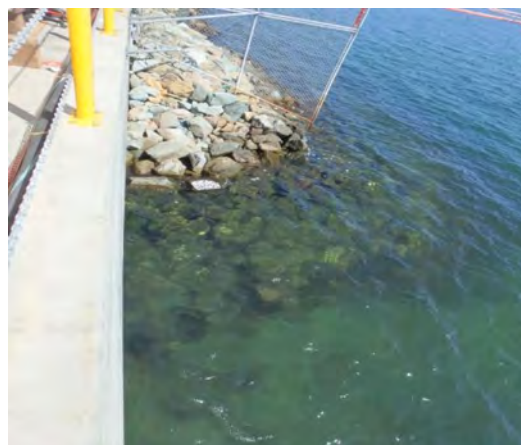
Subsurface and sloped revetment to be removed
