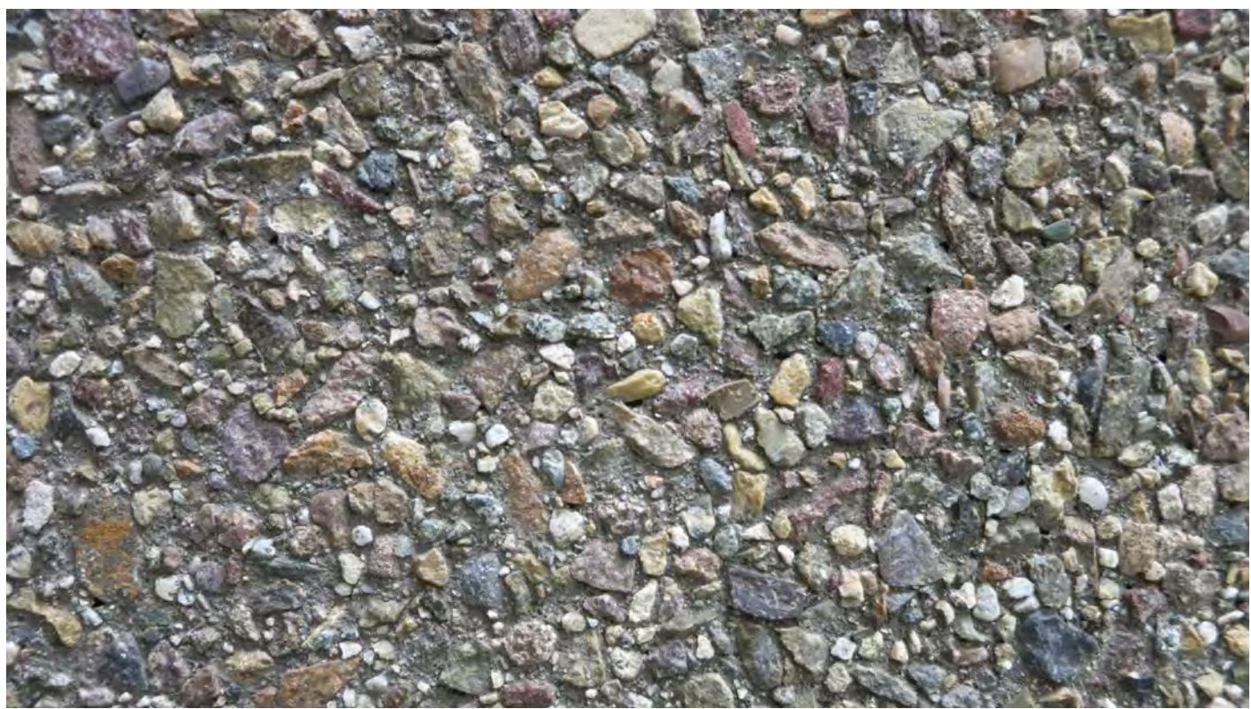
Paving Type 3: Promenade C.I.P. concrete Integral color, exposed aggregate finish
