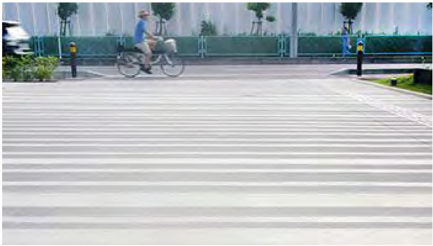
Paving Type 4: Delineated Path C.I.P. concrete Integral color, top cast finish, enhanced score patterning
