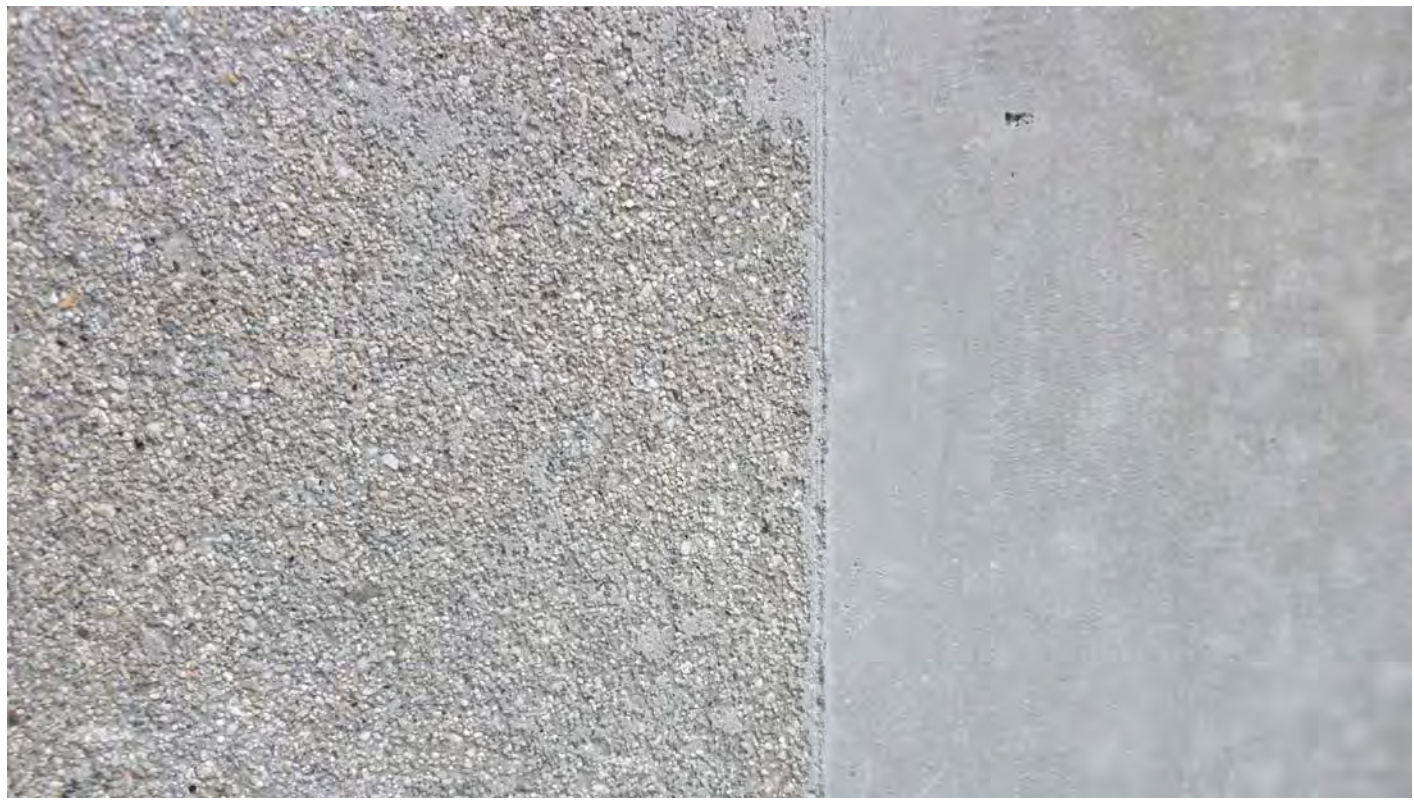
Paving Type 2: Bay to Street Connections C.I.P. concrete Integral color, top cast finish
