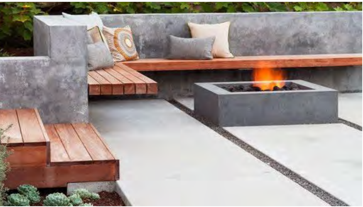
Bench C.I.P. concrete forms, wood-topped seating
