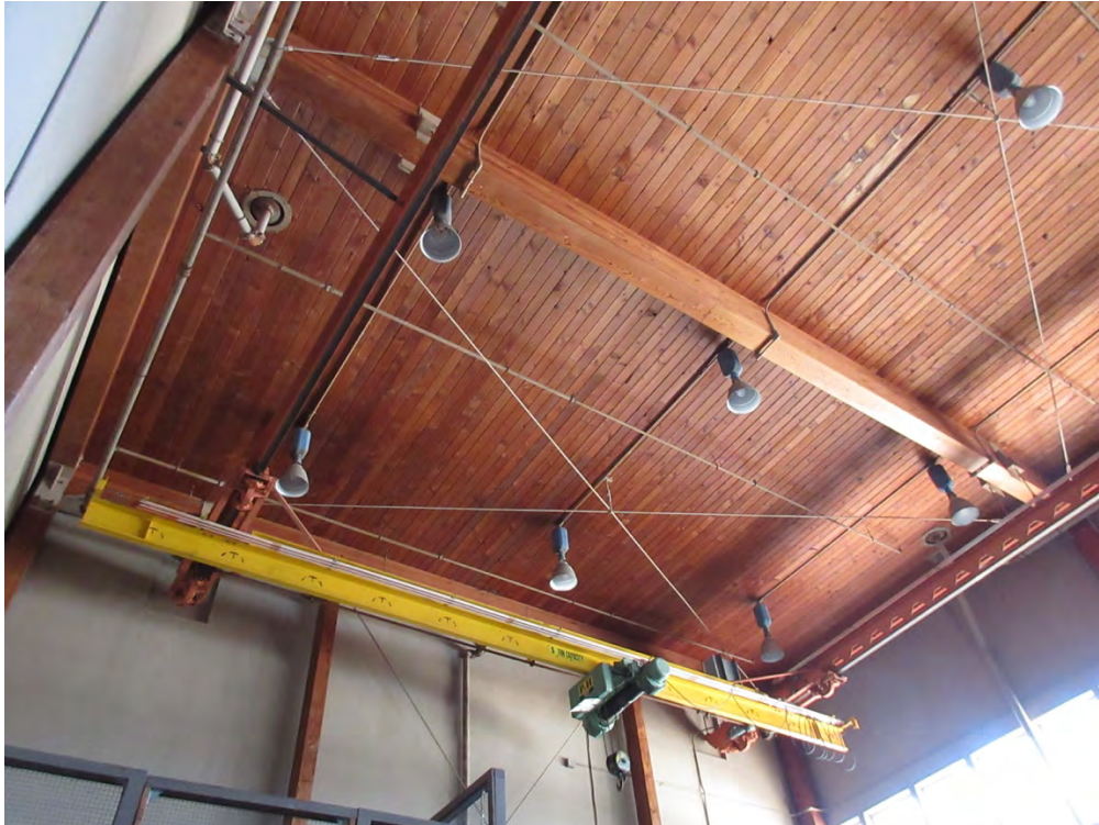
Photo 23: Maintenance Shop, exposed wood ceiling, work lights, and 5-ton hoist, looking northwest.
