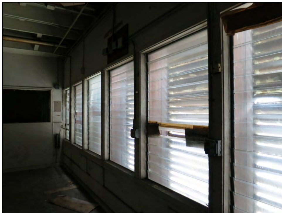
Figure 42. Jalousie windows in south machine shop.
