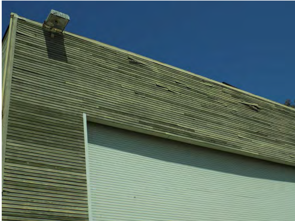
Photo 9 – Loose Shiplap Siding
