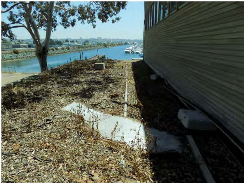
Photo 10 – Soil and root growth on North Roof
