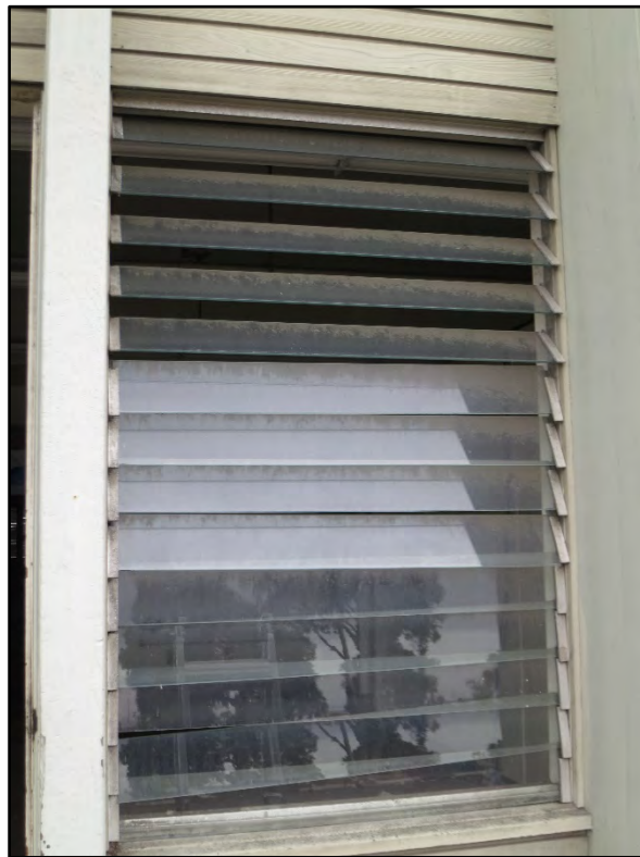
Figure 33. Detail of jalousie window on north façade.
