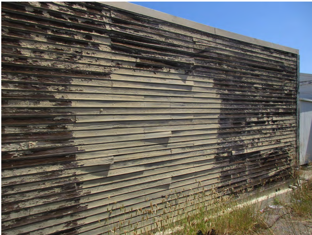
Photo 12: South façade showing warped and weathered redwood siding, looking northeast.
