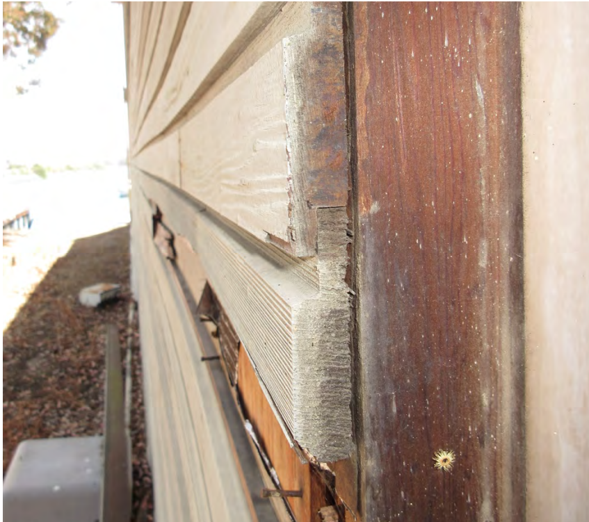
Photo 13: End view of the T&G redwood siding, looking east.
