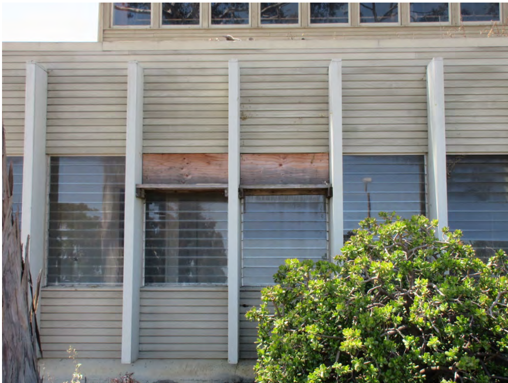
Photo 14: Detail of the north jalousie-style office windows and shade fins, looking south.
