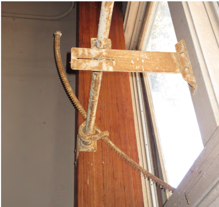
Photo 24: Detail of the opening mechanism for the clerestory windows. All windows open together.
