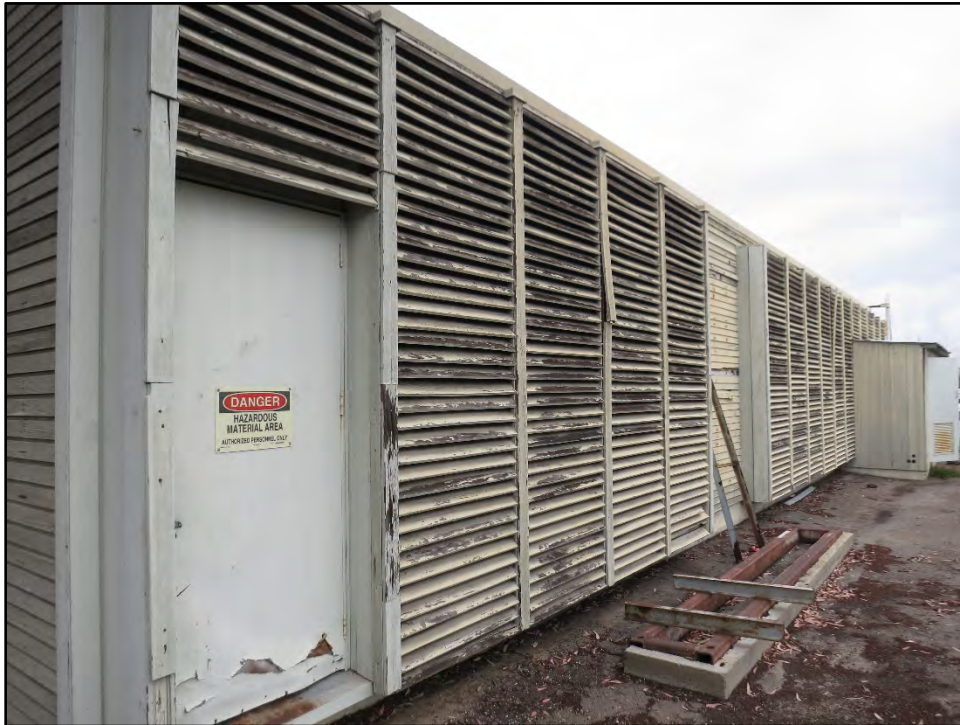
Figure 26. Redwood louvers on south façade.
