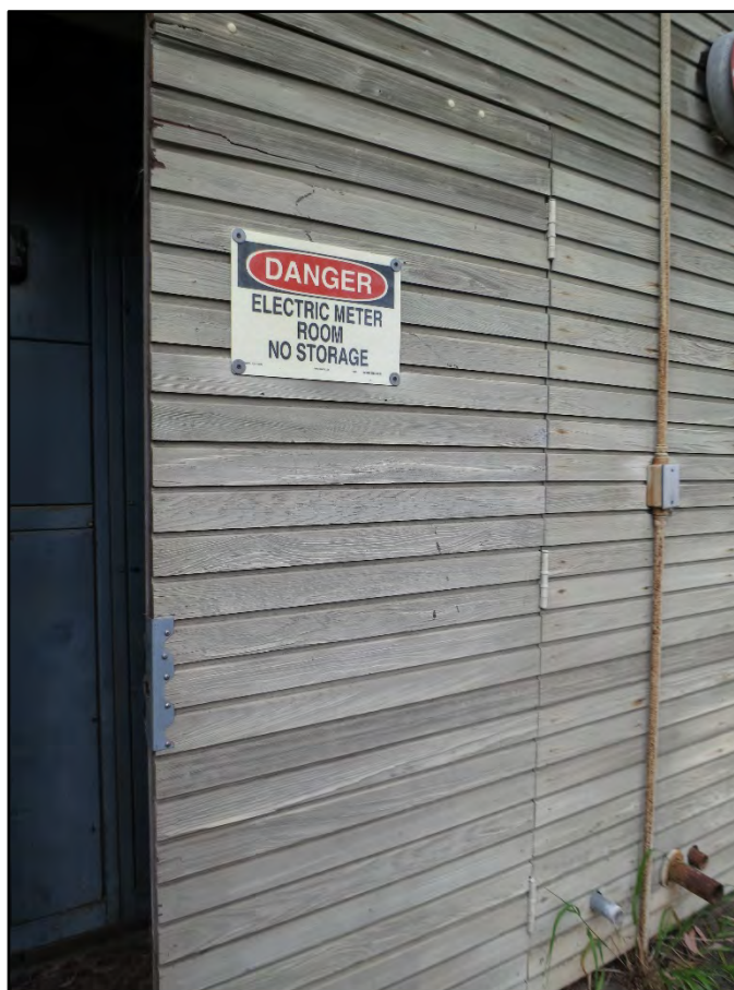
Figure 23. Door hidden by cladding on west façade.
