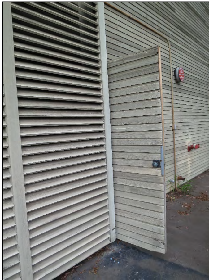
Figure 24. Detail of hidden door and redwood louvers on west façade.
