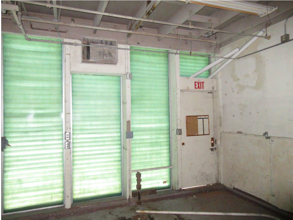
Photo 27: Shop wing, looking south. The green fiberglass panels are not original.
