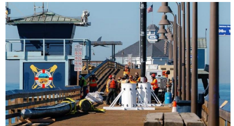
Pier Utility Repairs and Pile Replacement in Imperial Beach
