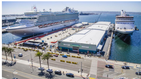
The Curtain Wall Repairs and Stormwater Improvements at B Street Pier in San Diego
